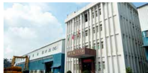
Pipe and Tube Mill
