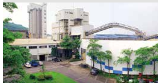
The slag powder grinding plant in Kaohsiung
