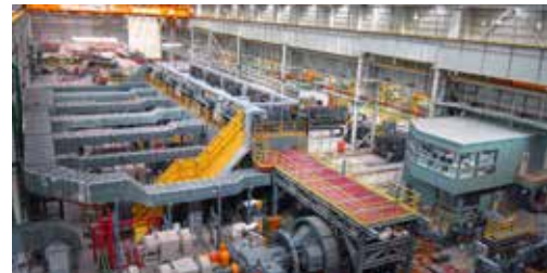
Mechanical and electrical equipment installation and maintenance
