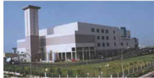
Refuse incineration plant engineering
