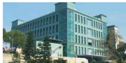
Biopharmaceutical plant engineering
