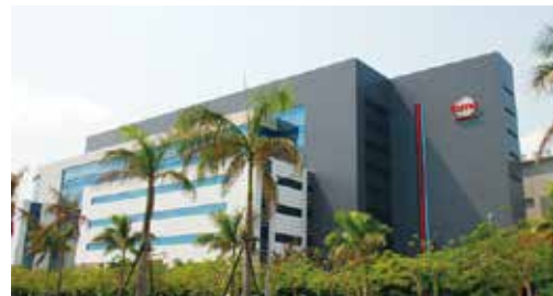
Plant building for TSMC
