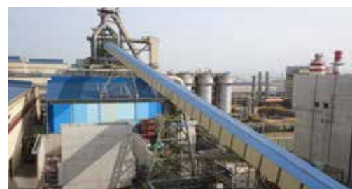
Manufacture and erection of DSC's blast furnace
