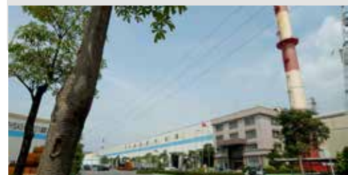
Hot Rolling Mill
