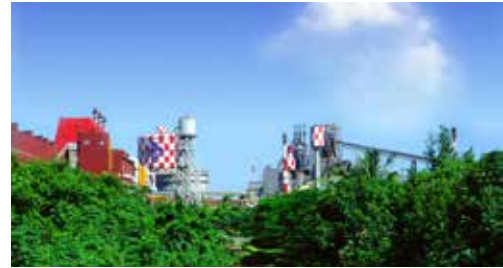
Greening inside the plant
