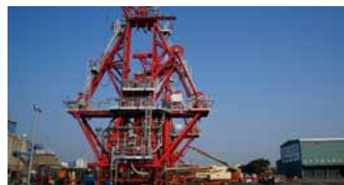
Manufacture and erection of the Crown mounted compensator
