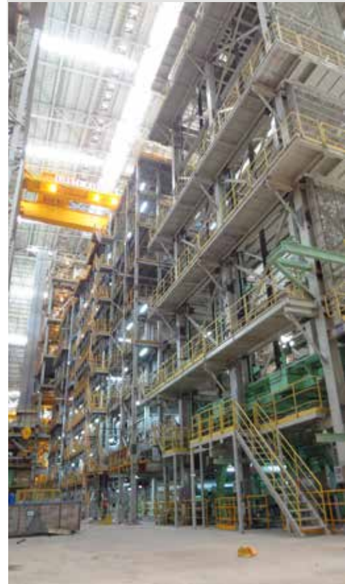
A Continuous Galvanizing Production Line
