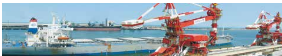
Manufacture and erection of DSC's continuous ship unloading equipment
