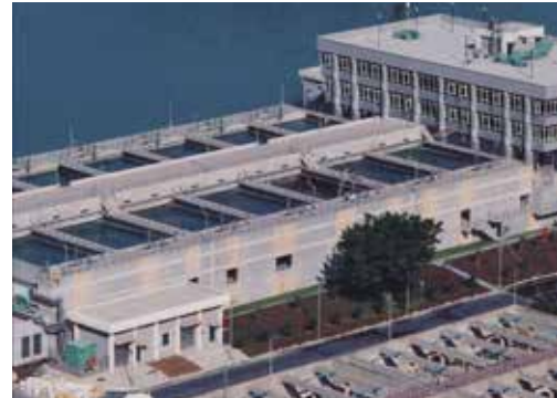
Advanced water purification engineering
