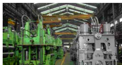
Manufacture and erection of CSC's and DSC's continuous casters
